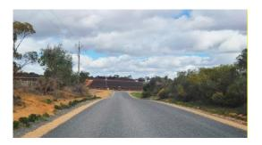
Both of these roads have been upgraded from having a sheeted surface to a 6.2 metre two coat spray sealed surface to improve the road ride quality and reduce long term road maintenance costs associated with unsealed roads.
